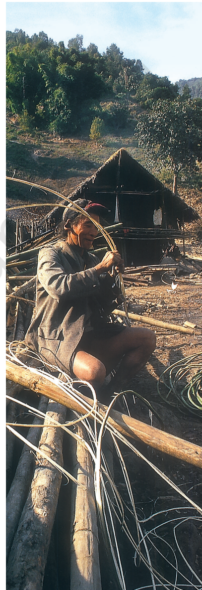
Fig. 5 – A log house being built in a village of the Nyishi tribes of Arunachal Pradesh.
